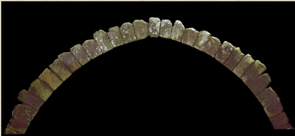
(b) Upstream view of one slice upon the arch showing diversity of the stones shapes and position of the real contact interfaces
