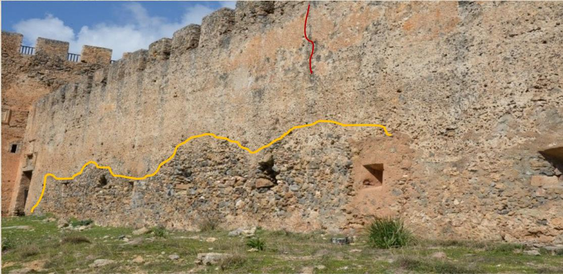
Disruption of the masonry, on the lower level of a south wall
